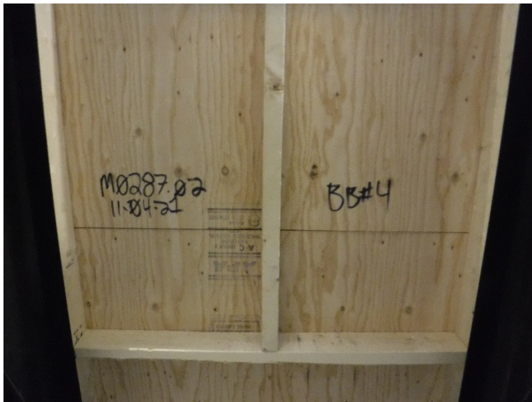
Photo No. 22 TEST #4 Underdeck During Test
