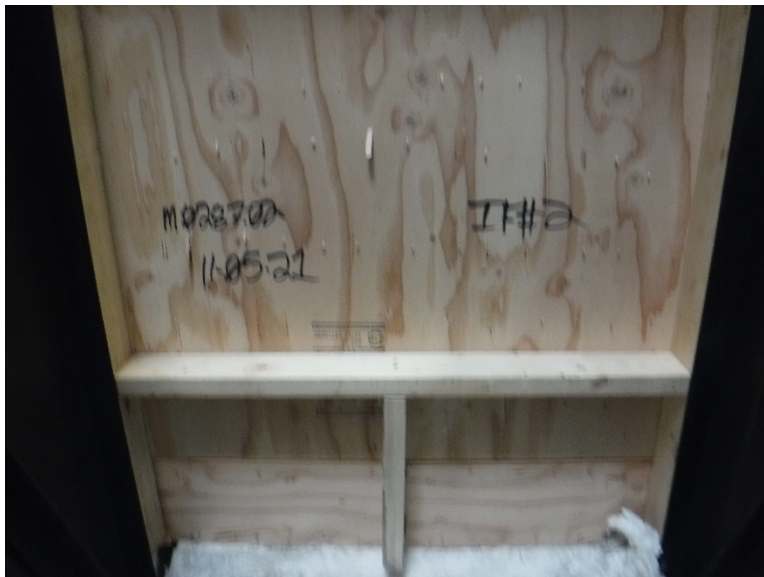
Photo No. 34 TEST #6 Underdeck During Test
